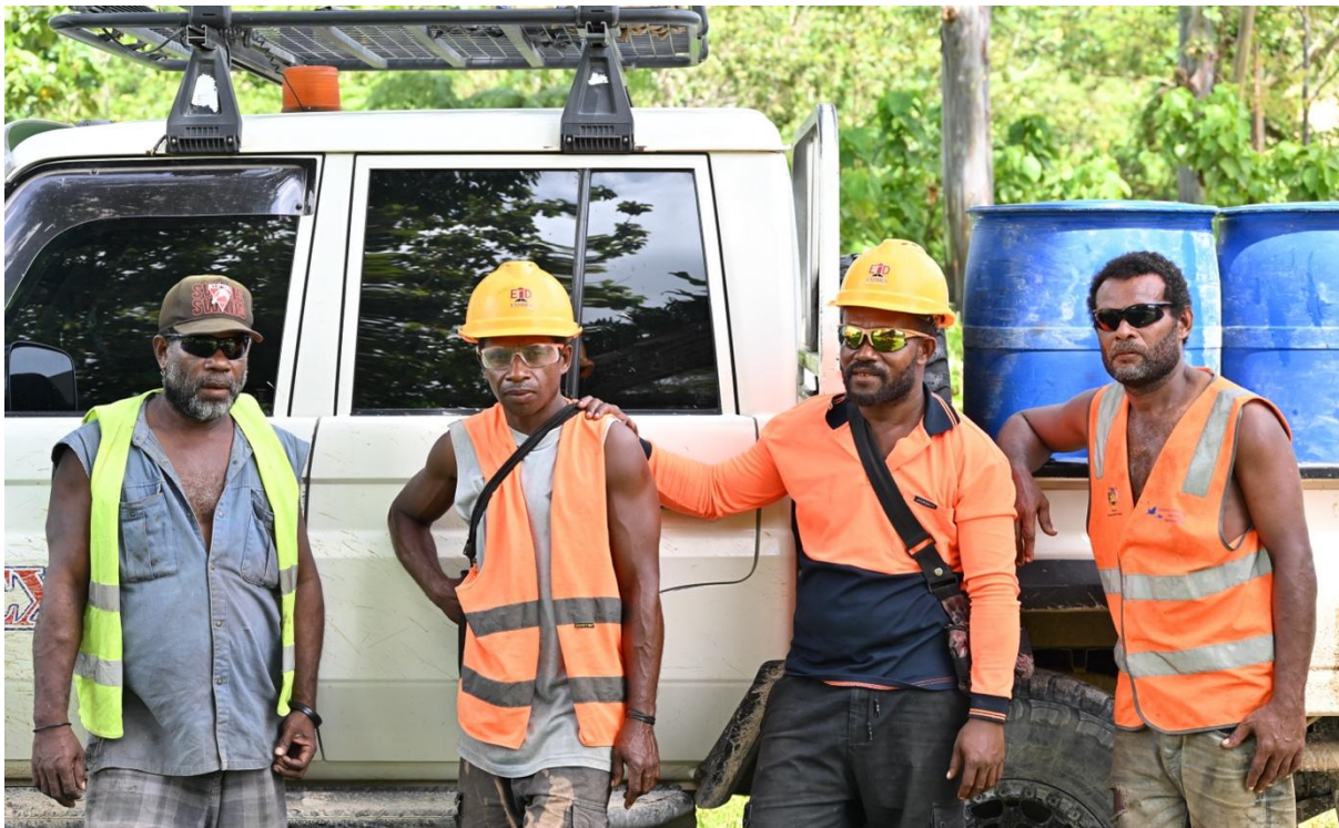
Photo 3 – The road works have been 100 percent delivered by Solomon Islanders, including those sourced from local communities.
